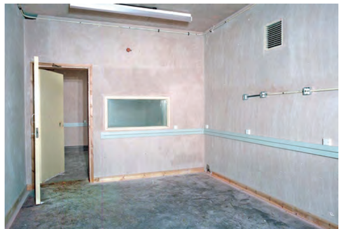
BBC office with a window into the BBC studio. The studio had sound insulation. The rest of the bunker could have been a noisy place with machinery and (probably frantic) people rushing around keeping track of nuclear bursts and enemy action. Photo Nick Catford
